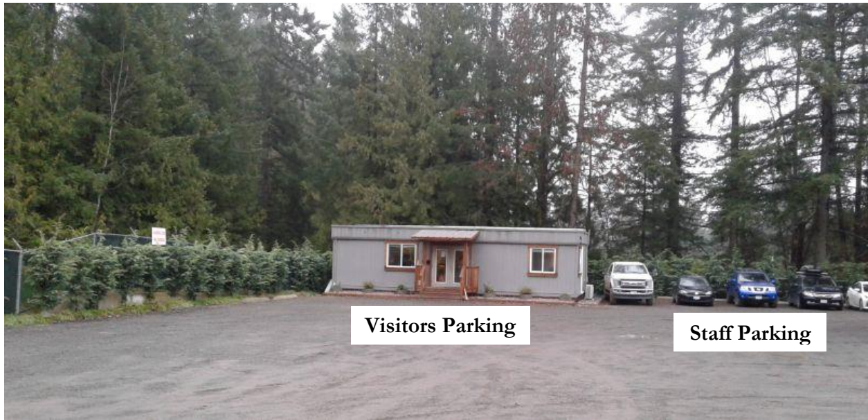
Figure 7: Location of the Northern Building
