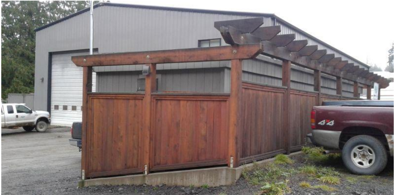
Figure 9: Solid Wooden Fencing to Shield the Southern Building
