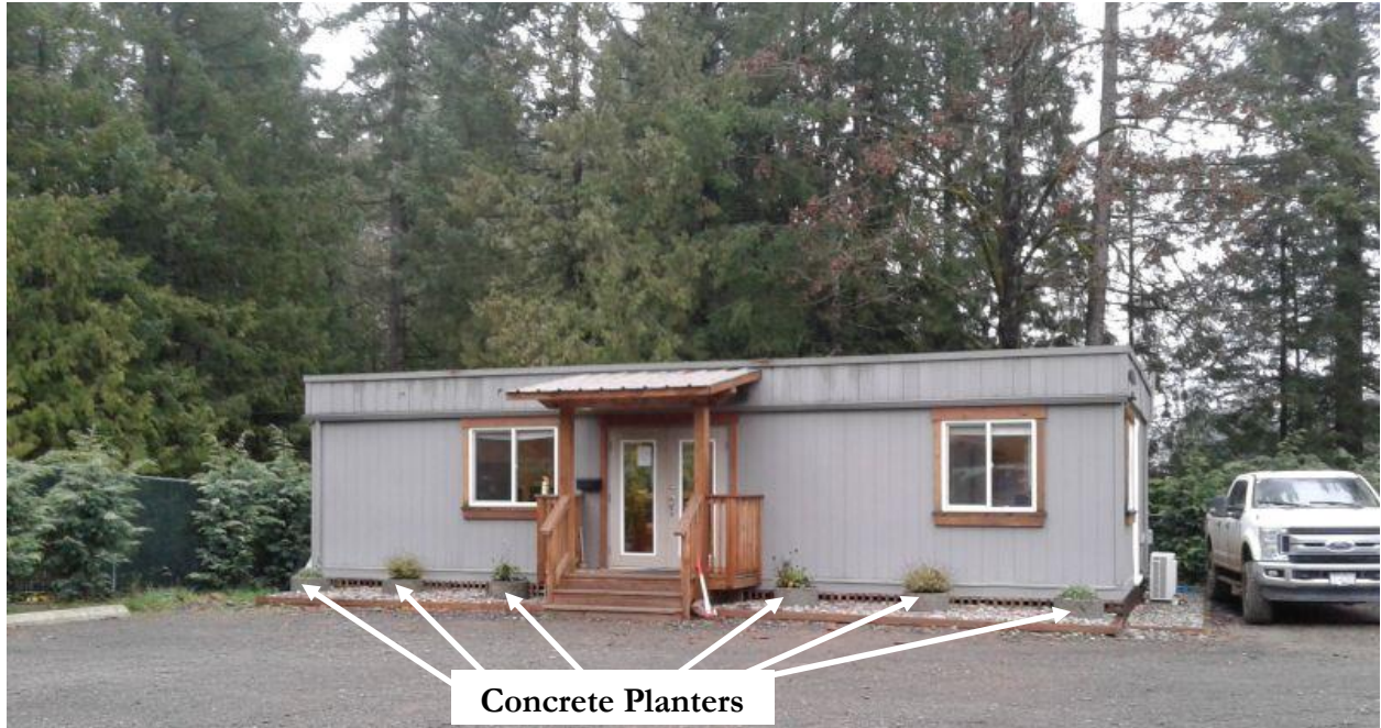
Figure 5: Northern Building Used as Administrative Office
