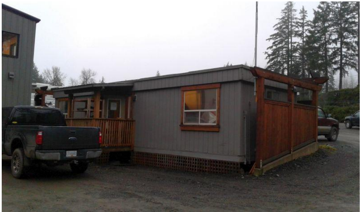
Figure 6: Southern Building Used as Crew Office
